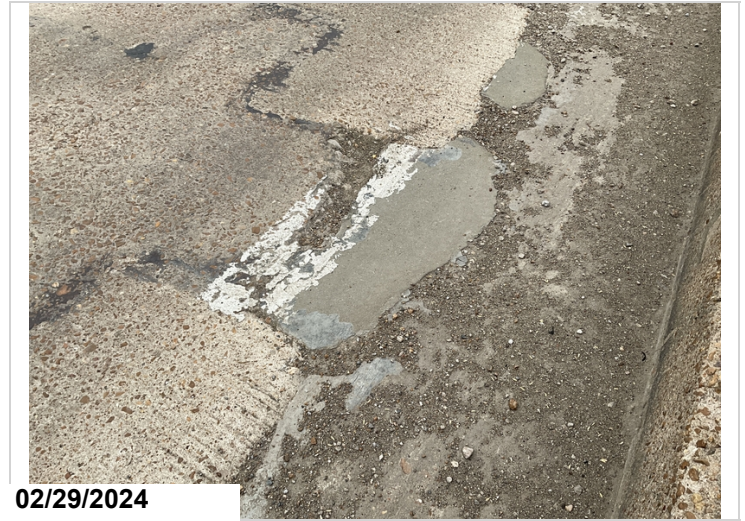
Span 3, right lane has spall next to shoulder. CS3
