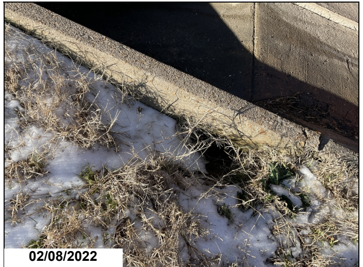
Bent 5 slope near top both sides have holes going under concrete slope.
