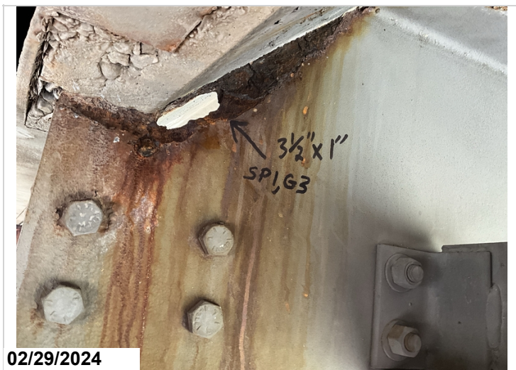
Span 1, bent 2, girder 3 in haunch area has a 3 1/2"x1 1/2" hole. CS3
