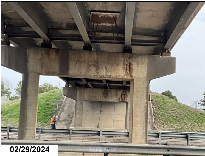
Bent 3, lower ahead face has large longitudinal cracking, and large spalled area above column 1. Both defects CS3
