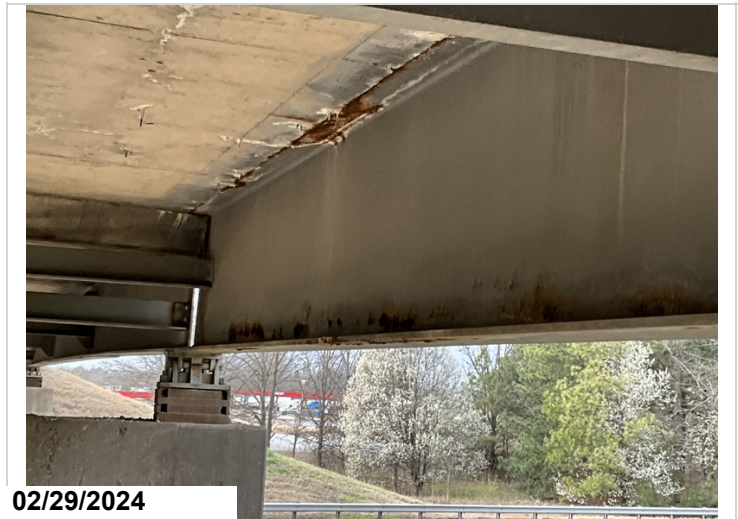
Span 1 girder 5 has active corrosion to top flange and bottom flange area.
