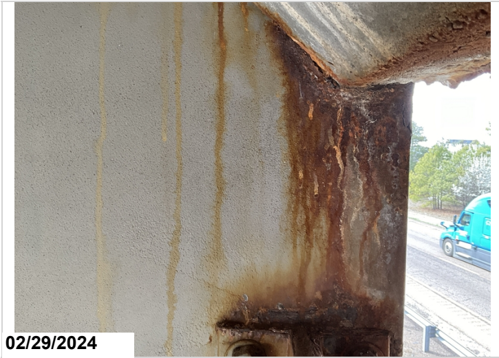
Span 3, bent 3, girder 5 in the haunch area has up to 1/8" section loss. CS3
