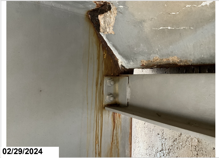
Abutment 1 girder 5 at haunch area has active corrosion with section loss. 1/16". CS3
