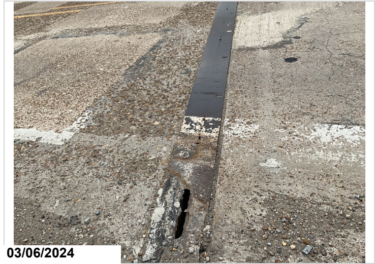
Bent 3 assembly joint has holes rusted 10' CS4: 3' CS3
