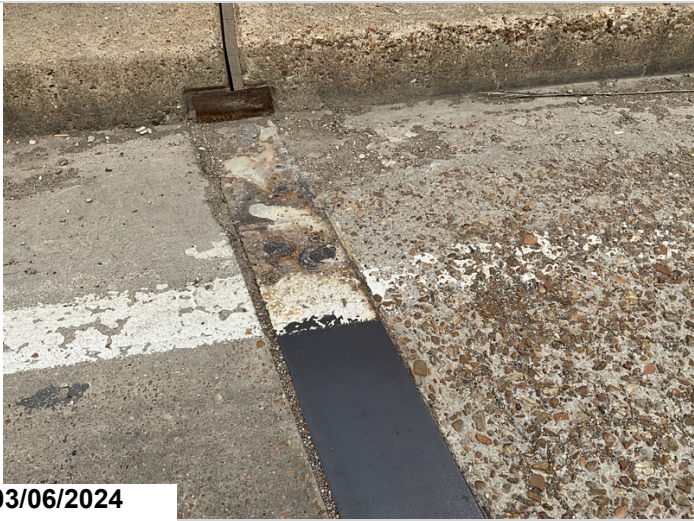
Bent 4 right side assembly joint has corrosion with heavy section loss. Both shoulders CS3
