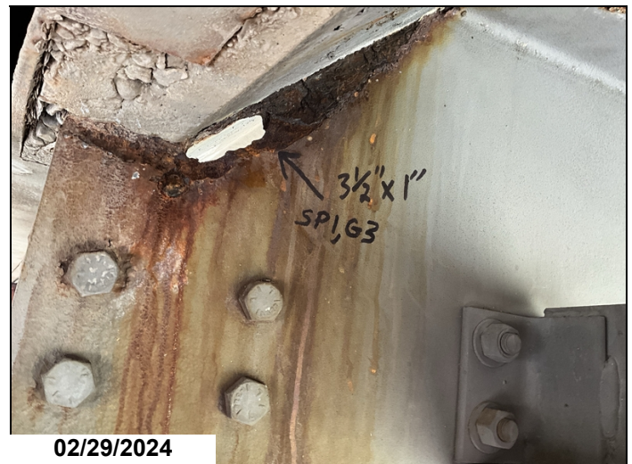
Span 1, bent 2, girder 3 in haunch area has a 3½"x1" hole. CS3
