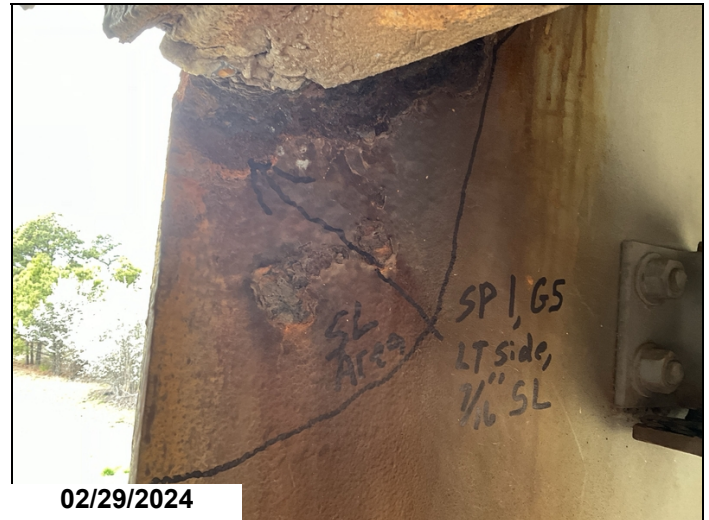
Span 1, bent 2, girder 5 in the haunch area has up to 7/16" section loss. CS3
