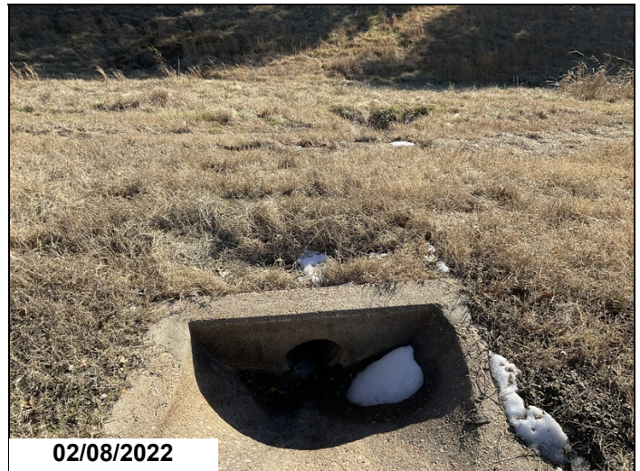
Bent 5, left side drain is broken and washing out slope.
