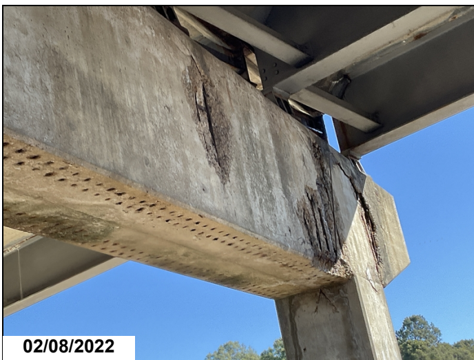
Bent #2 ahead face cap
