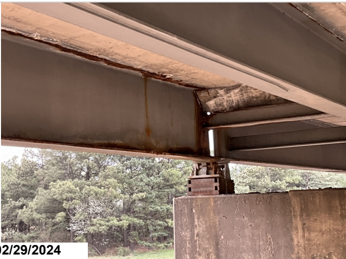
Span 1 girder 1 has flaking rust to the top and bottom flange.
