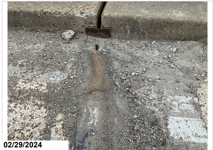
Bent 2 assembly joint has holes rusted on both shoulders. CS4 2': CS3 2' corrosion.
