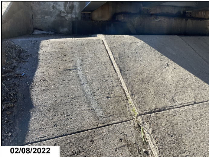
Bent 5, left slope pavement has settled 2".
