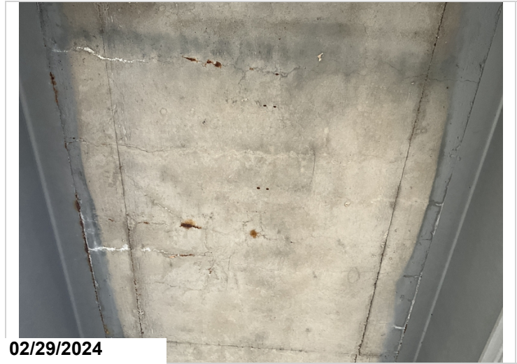
Span 4, bay 1 has efflorescent leaching with rust staining. CS3
