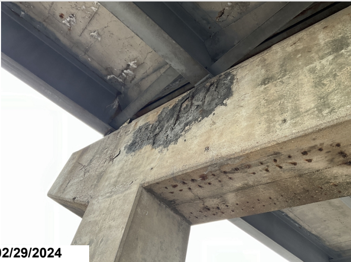
Bent 4 cap, backside, above column 1 has large spalled area with exposed reinforcing steel with section loss. CS3
