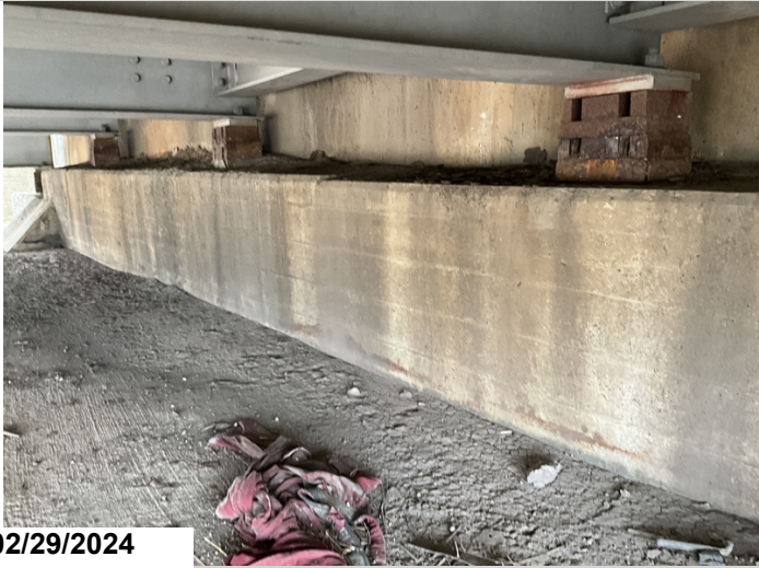
Bent 5 typical condition of fixed bearings. CS3
