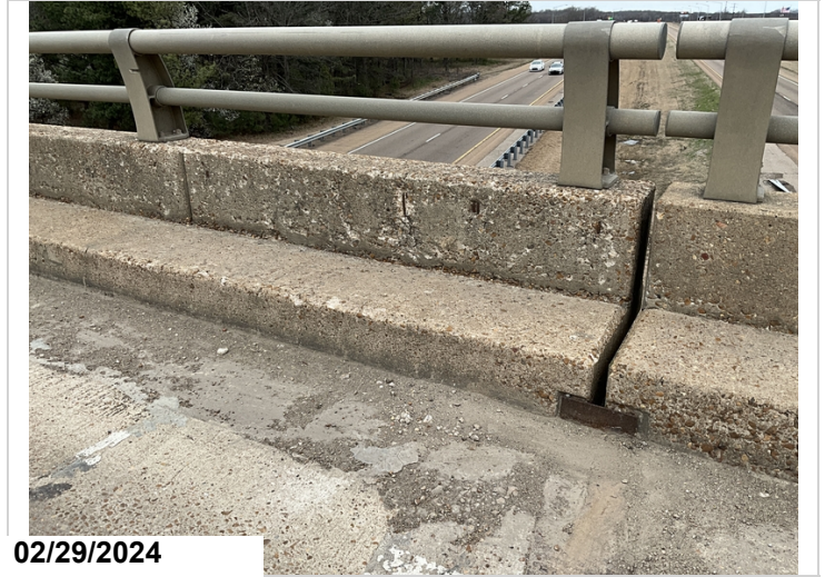
Span 3 right side has spalls with exposed reinforcing steel with no section loss. CS3 Spalling
