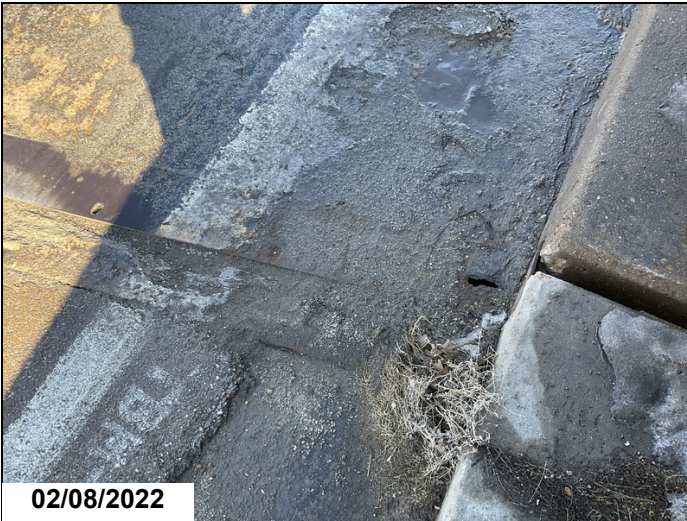
Bent #5 left shoulder top plate has a 4" area with 100% section loss.
