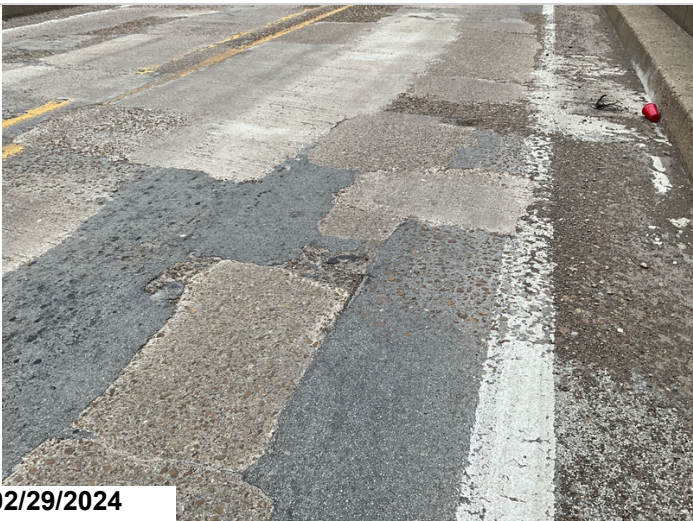
Span 1, right lane has shallow spalled areas. CS3
