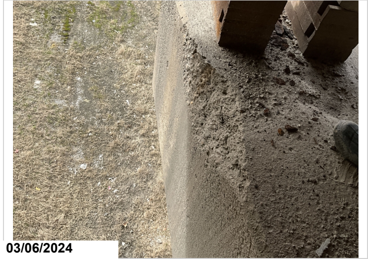
Bent 3 ahead, right side has large spall near bearing area. CS3
