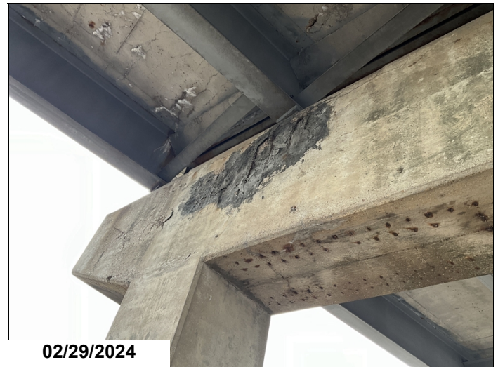
Bent 4, backside, above column 1 has large spalled area with exposed reinforcing steel with section loss. CS3
