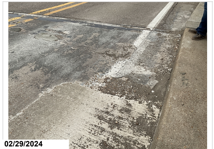
Span 4, right lane has large spalls . CS3
