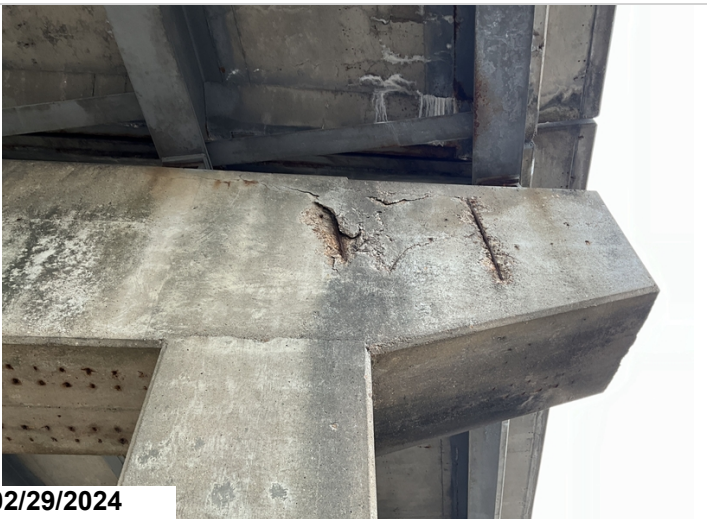
Bent 4, backside, above column 2 has large spalled area with exposed reinforcing steel with section loss. CS3
