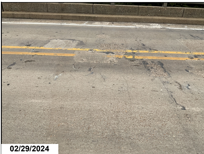
Span 4 has scattered areas of spalls/delam. CS3
