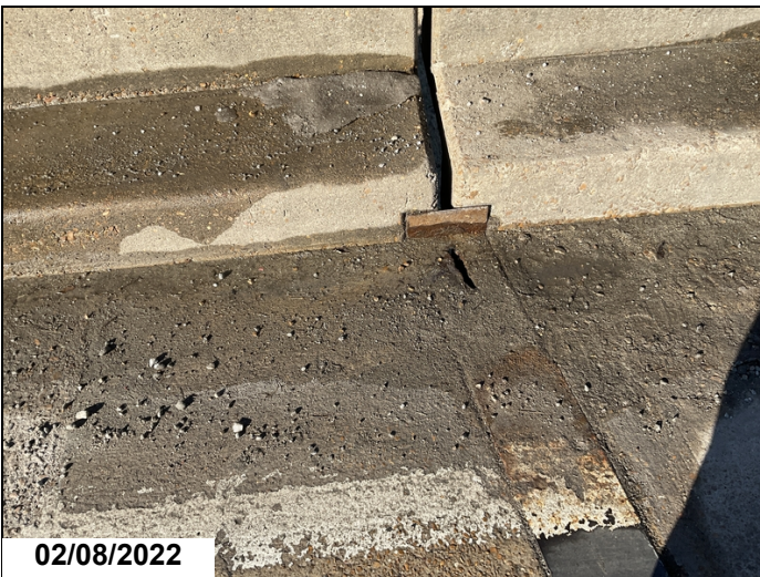
Bent #2 right shoulder top plate has a 6" area with 100% section loss.
