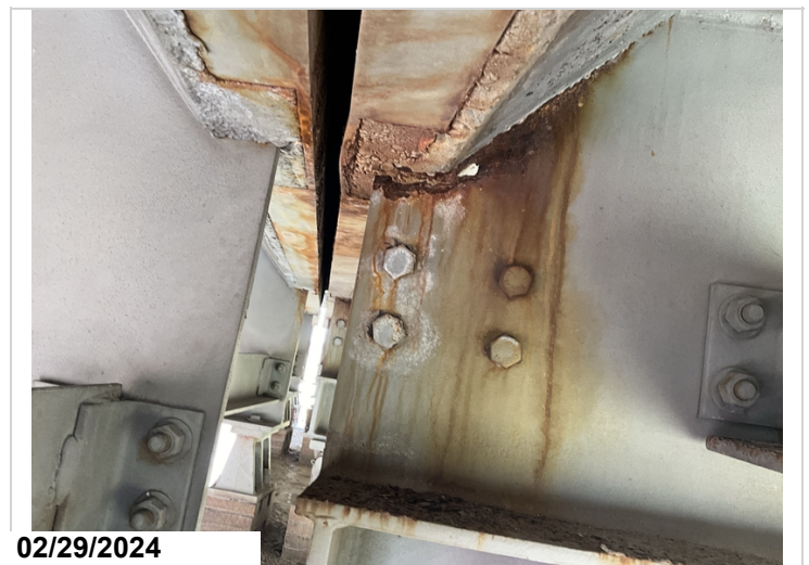
Span 1, bent 2, girder 2 has a hole in the haunch area 1"x5". CS3
