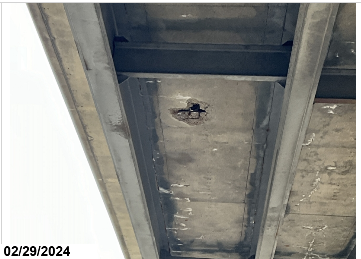
Span 3, bay 4 has large spall with reinforcing steel exposed with section loss. CS3
