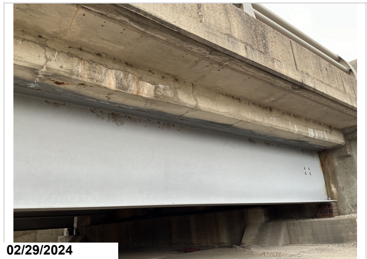
Span 4, Bent 5, right side deck has efflorescent leaching. CS3
