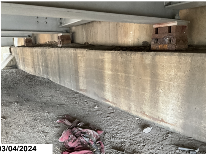
Bent 5 typical condition of fixed bearings. CS3 This is typical condition of all bearings
