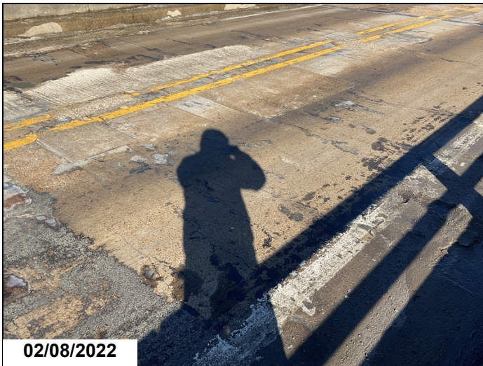
Typical deck cracks.
