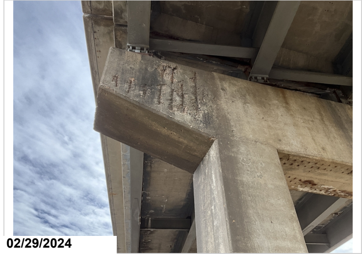
Bent 3 back has large area with exposed reinforcing steel with section loss. CS3
