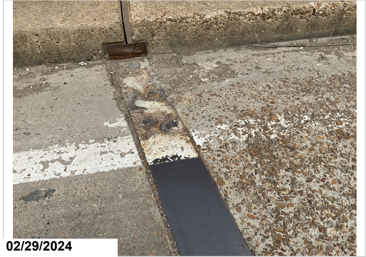
Bent 4 right side assembly joint has corrosion with heavy section loss. Both shoulders CS3
