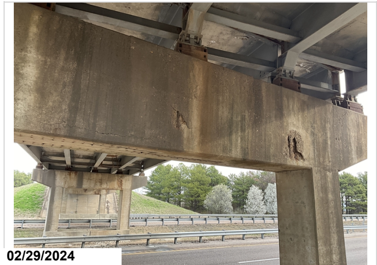
Bent 4, ahead has large spalls with exposed reinforcing steel with section loss. CS3
