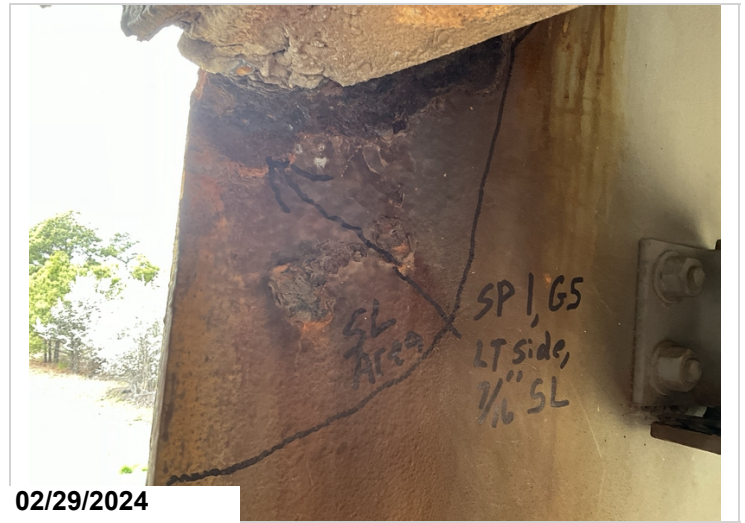
Span 1, bent 2, girder 5 in the haunch area has up to 7/16" section loss. CS3
