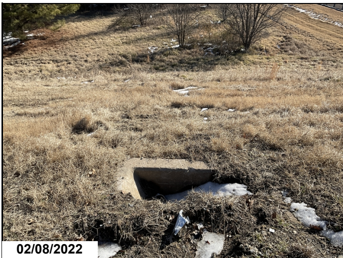
Bent 1, left side drain stopped up pipe and has been disconnected.
