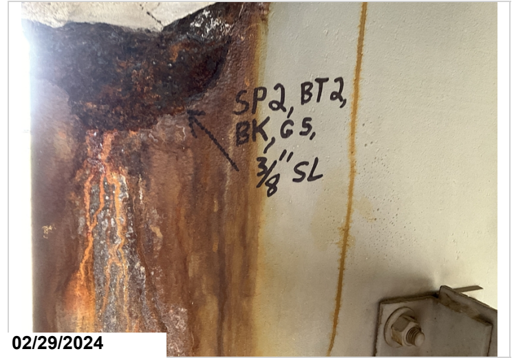
Span 2, bent 3, girder 5, in haunch area has up to 3/8" section loss. CS3
