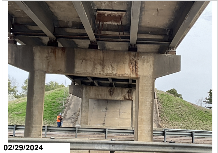
Bent 3, lower ahead face has large longitudinal cracking, and large spalled area above column 1. Both defects CS3
