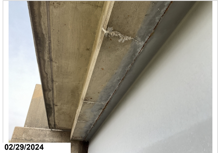
Span 1, right soffit area has heavy leaching to deck. CS3
