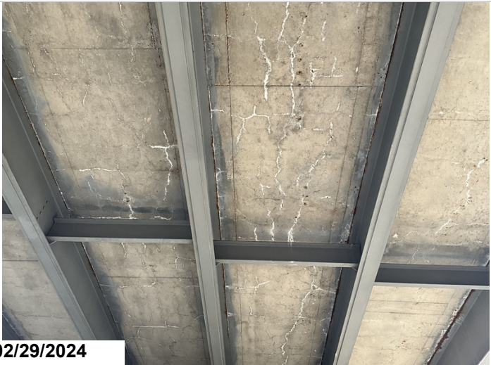
Span 1 under surface showing heavy leaching throughout. CS3
