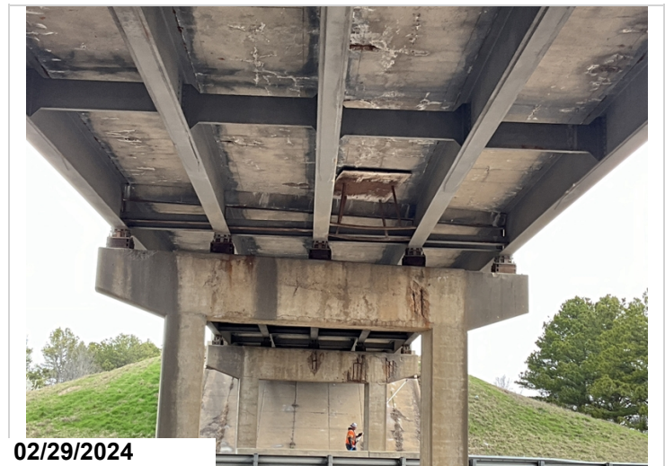
Bent 3, ahead, span 3 , bay 2 has full depth repaired area.
