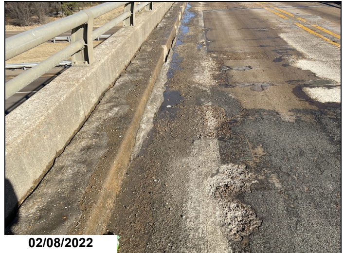
Span #4 has 20 square feet of shallow spalling near or in gutters.
