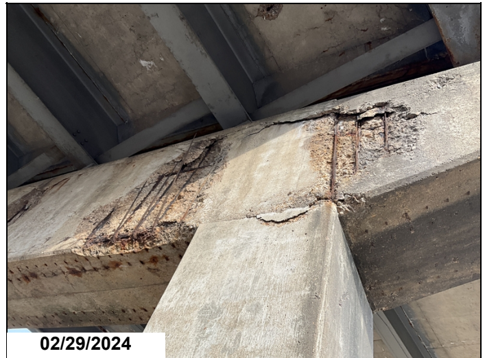
Bent 2 ahead has large area of exposed reinforcing steel with heavy section loss to rebar. CS3
