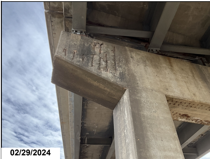
Span 2 bent 3 back has large area with exposed reinforcing steel with section loss.
