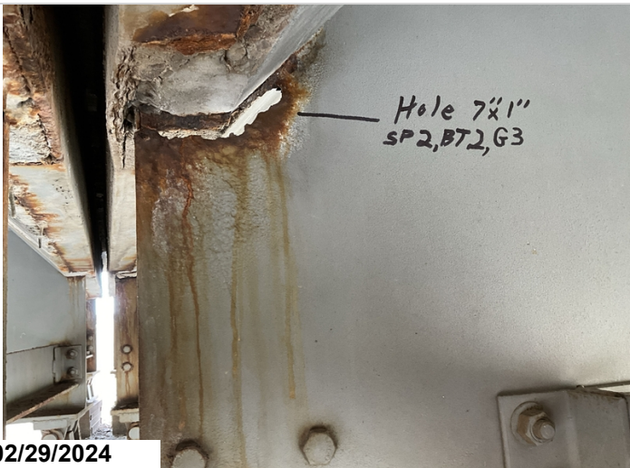
Span 2, bent 3, girder 3, haunch area has a 7"x1" hole. CS3
