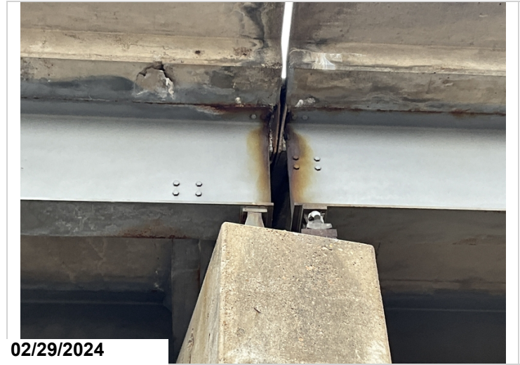
Bent 3 girders 5 has surface corrosion with minor section loss to end of girder. 1/16" CS3
