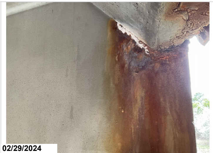
Span 2, bent 2, girder 5, in haunch area has up to 1/8" section loss. CS3
