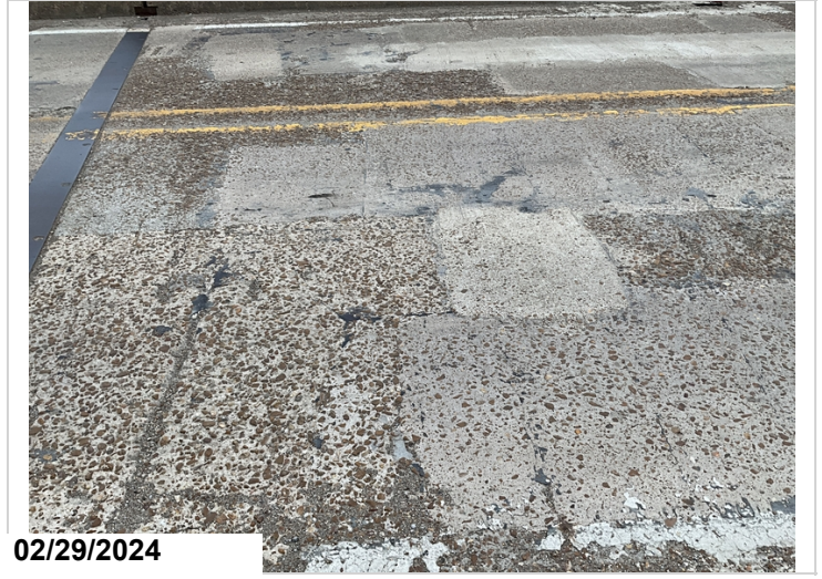
Span 1, left lane has sealed and a few unsealed transverse cracks. CS3
