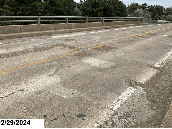
Typical photo of span 3. CS3 Abrasion
