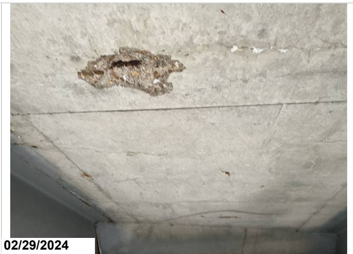
Span 4, bay 1 has spalling with exposed reinforcing steel with section loss. CS3
