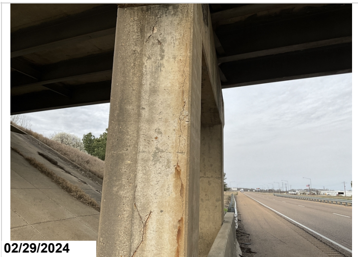
Bent 4, column 1, left side has vertical crack with rust staining. CS3
