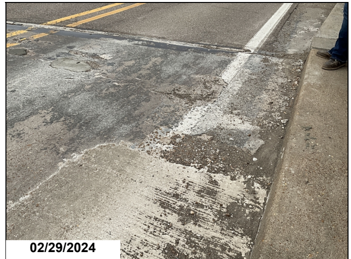
Span 4, right lane has large spalls . CS3
