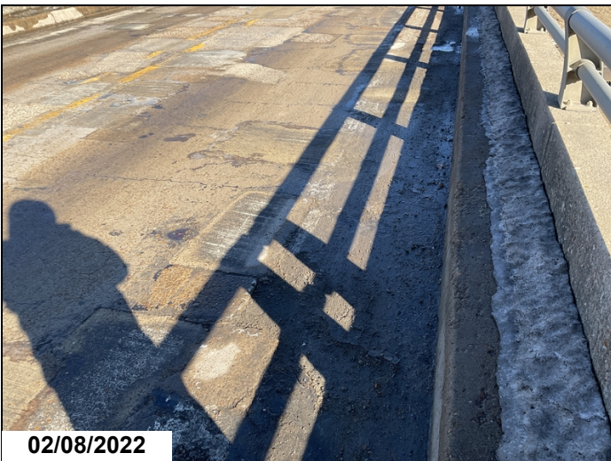
Span #3 has 8 square feet of small spalls with no rebar exposed.
