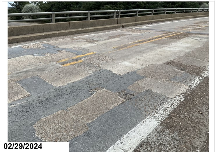
Span 1, typical photo of deck patches sound and unsound patches.
