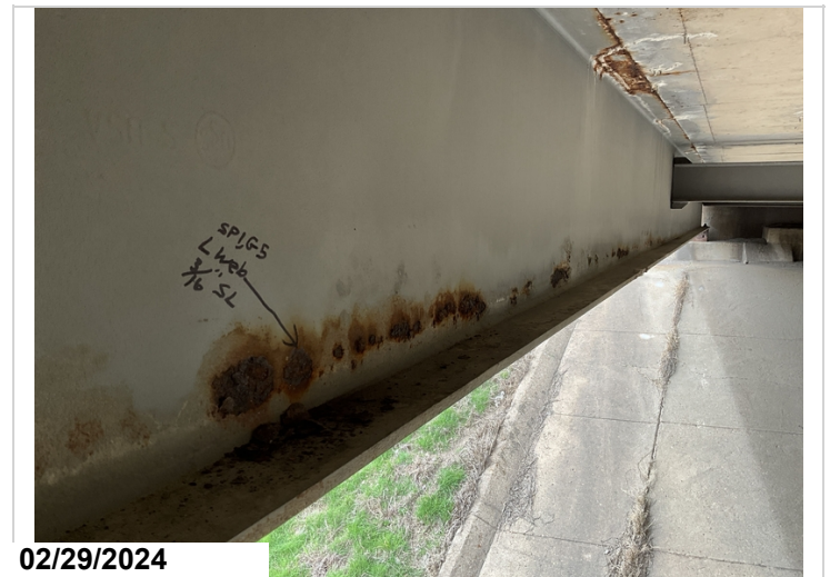
Span 1, girder 5, 5' back of bent 2, has areas with up to 3/16" section loss at mid span there are several other locations that appear to have the same amount of corrosion. CS3
