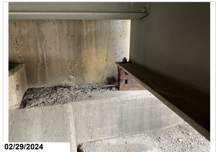
Bent 5, bay 4, vertical cracks. CS2
