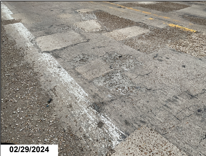
Span 2, left lane has large spalled areas. CS3
