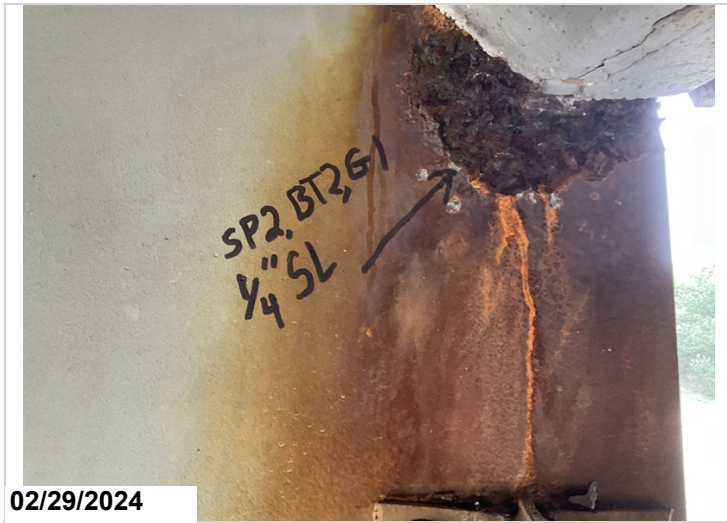
Span 2, bent 3, girder 1, in the haunch area has up to 1/4" section loss. CS3
