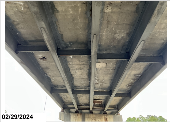
Span 3 has efflorescent leaching throughout at scattered locations. CS3
