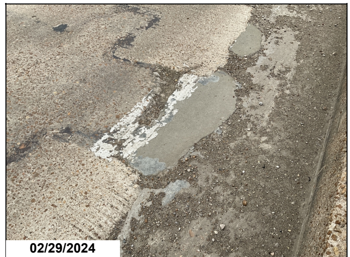
Span 3, right lane has spall next to shoulder. CS3
