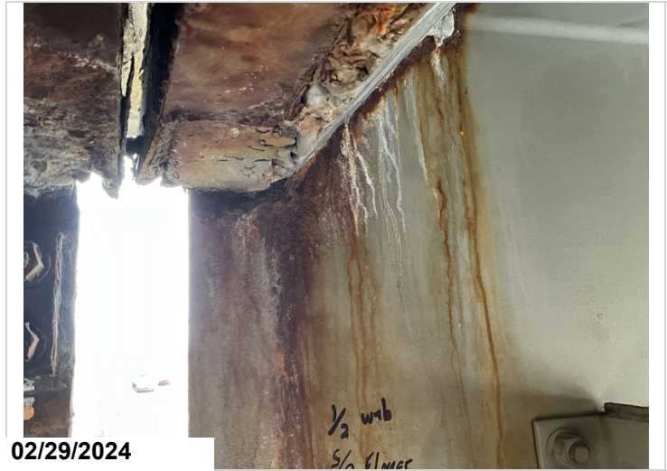
Span 2, bent 2, girder 1 in haunch area has up to 1/8" section loss. CS3
