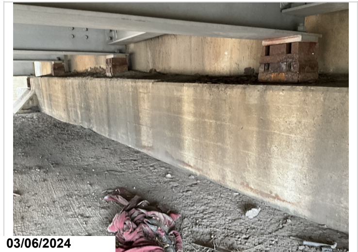
Bent 5 typical condition of fixed bearings. CS3 This is typical condition of all bearings
