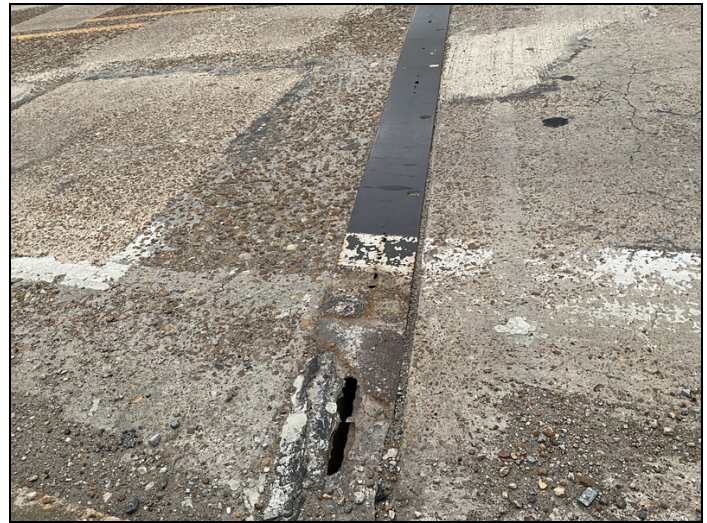
Bent 3 assembly joint has holes rusted 10' CS4: 3' CS3
