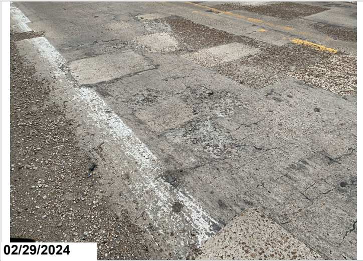
Span 2, left lane has large spalled areas. CS3
