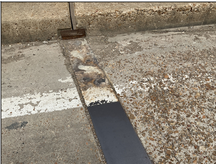
Bent 4 right side assembly joint has corrosion with heavy section loss. Both shoulders CS3
