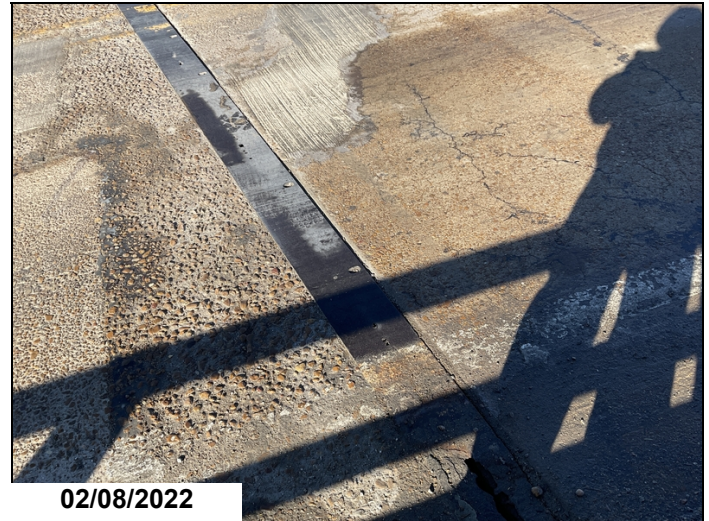
Bent #3 left shoulder top plate has a 6" long area and several small areas across joint with 100% section loss two feet total.
