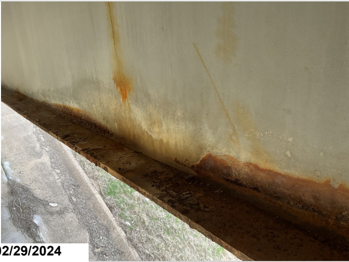
Span 1, bent 2, girder 1, bottom web flange juncture has section loss up to 15'. CS3
