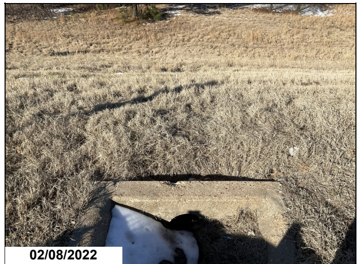
Bent 1, right side drain is broken and washing out slope.
