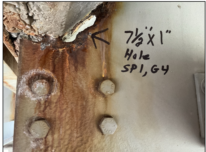
Span 1, Bent 2, girder 4 in haunch area has a 7 1/2"x1" hole. CS3
