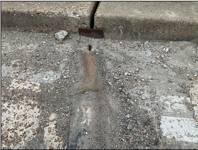
Bent 2 assembly joint has holes rusted on both shoulders. CS4 2': CS3 2' corrosion.
