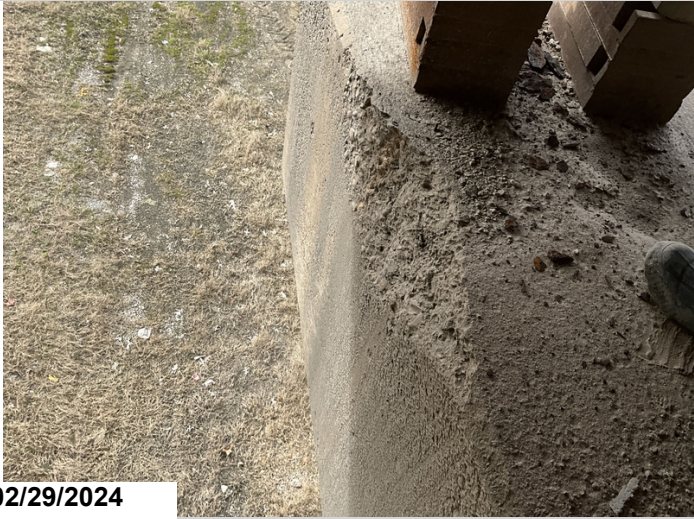
Bent 3 ahead, right side has large spall near bearing area. CS3
