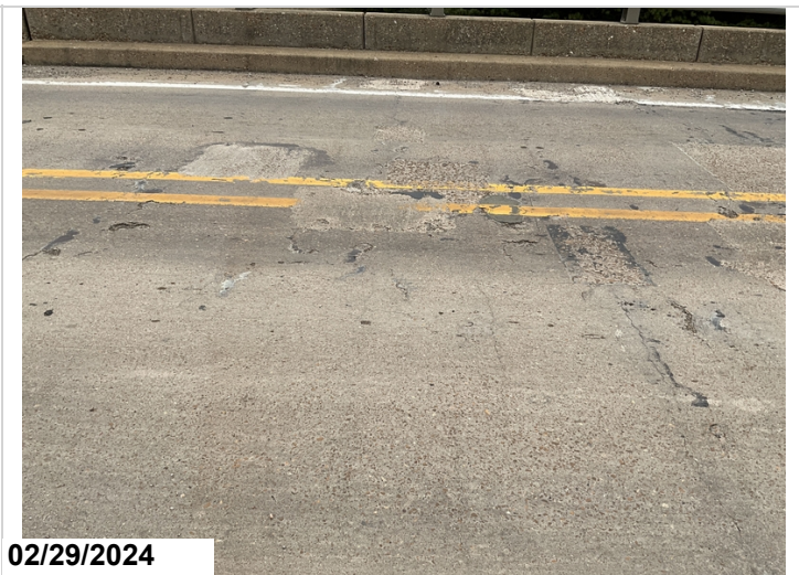
Span 4 has scattered areas of spalls/delam. CS3
