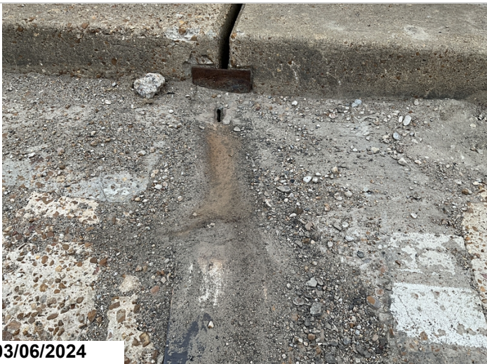
Bent 2 assembly joint has holes rusted on both shoulders. CS4 2': CS3 2' corrosion.
