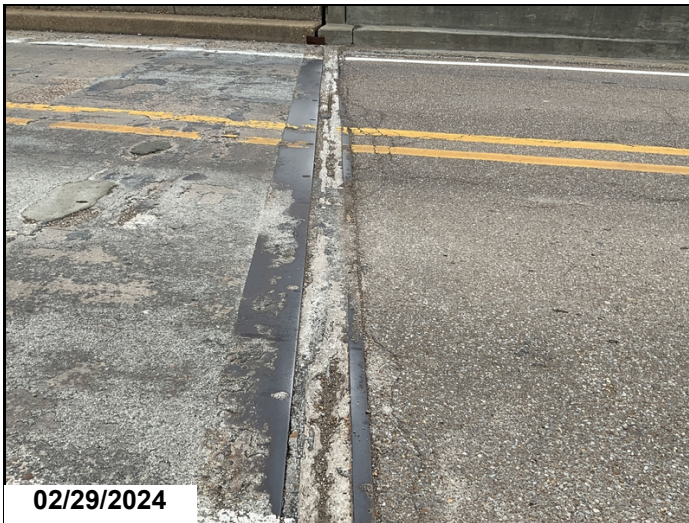
Bent 5 has spalling all the way across back wall, with exposed reinforcing steel in areas. CS3 Spalling, and exposed rebar.
